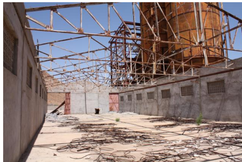
34a) Storage of packaged cement
