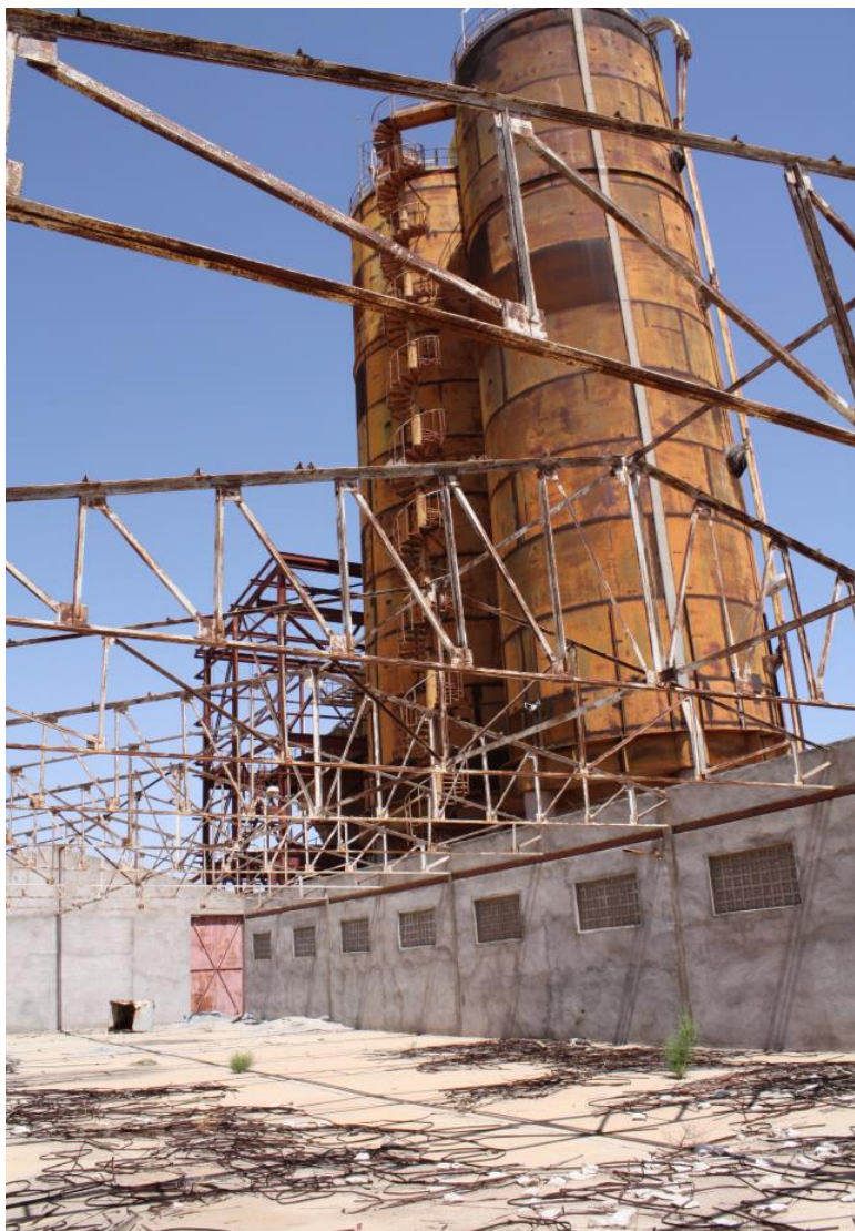
32) Transport and storage of the cement
